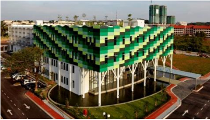
Image 2: NTT MSC Technology Center, a Malaysian ICT facility certified by the Green Building Index (Green Building Index, 2012)
