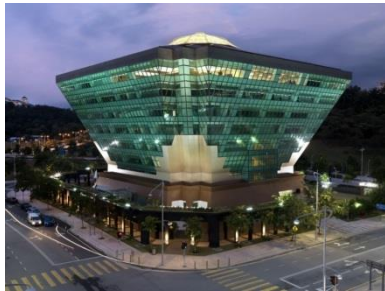
Image 1: Self shading and Dynamic shading system at ST Diamond Building
